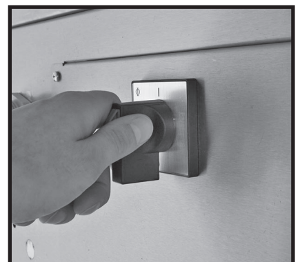
Switch off the main switch and close shut-off valve(s) at site.
